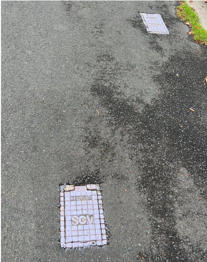
Figure 7. Typical examples of suitably coloured and labelled covers on network assets.
